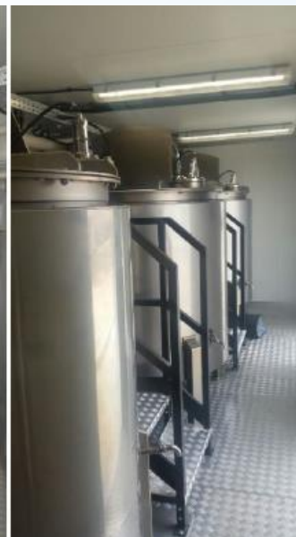
Neutralization of TMAH and N°3 bio-reactors in series
