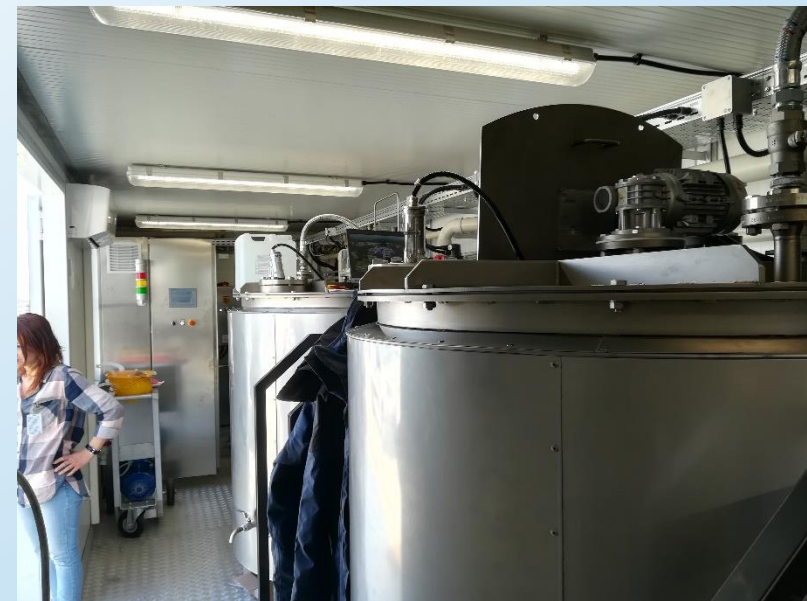
Neutralization of TMAH and N°3 bio-reactors in series
